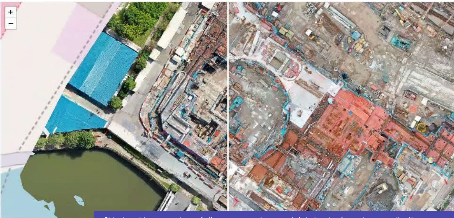
Side-by-side comparison of site progress using smart date tracker from drone application.
